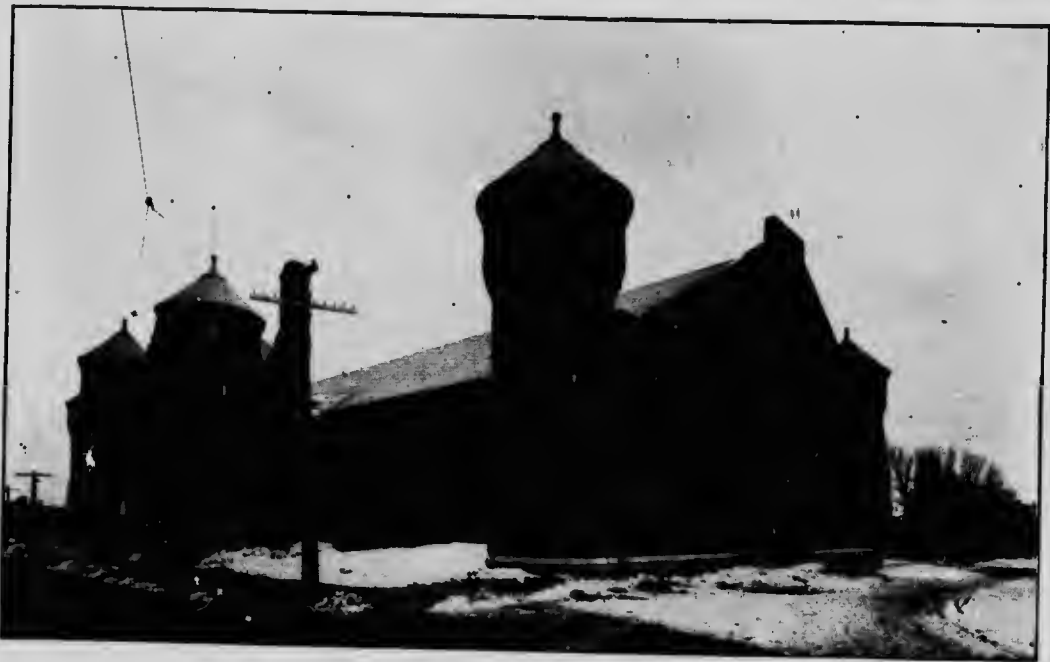
Brockville Drill Hall.
